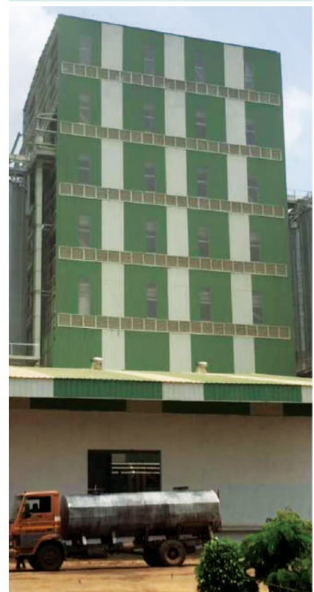
A view of feed mill
