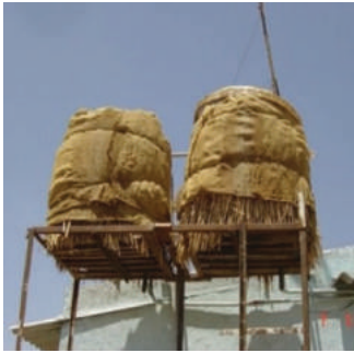
Fig-4:Insulation of tanks
