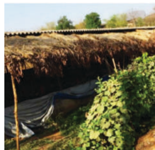
Fig-6: Insulation of roof-top
