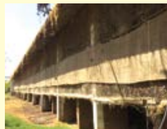
Side curtains to sheds
